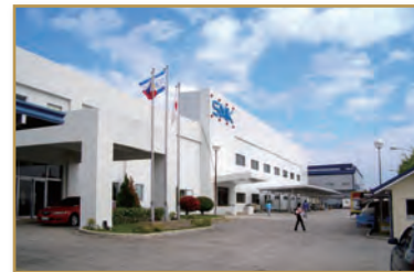
The Philippines factory after completion of expansion work
