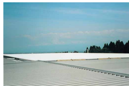
Rooftop after application of the coat for insulation against solar heat.
