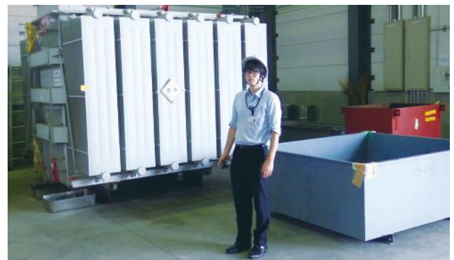
Inspection of PCB waste disposal site (Head Office)
